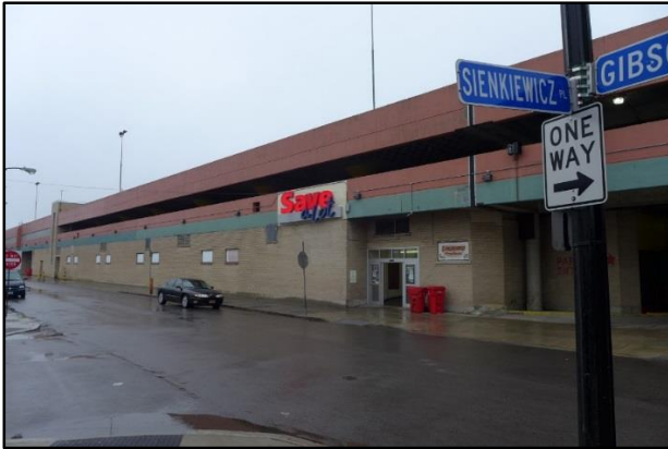
Gibson Street façade of Broadway Market
